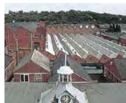
NSK Newark Plant
