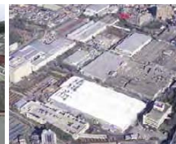
NSK Fujisawa Plant
